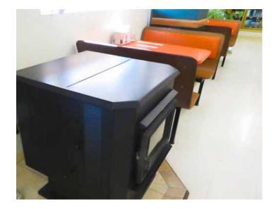
Solid-fuel burning appliances should be vented into a factory-built chimney tested and approved to UL 103 or UL 103 HT Standards; or a clay tile-lined masonry chimney.
